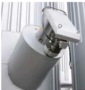
Figure 9: Stirring device on a bitumen tank
