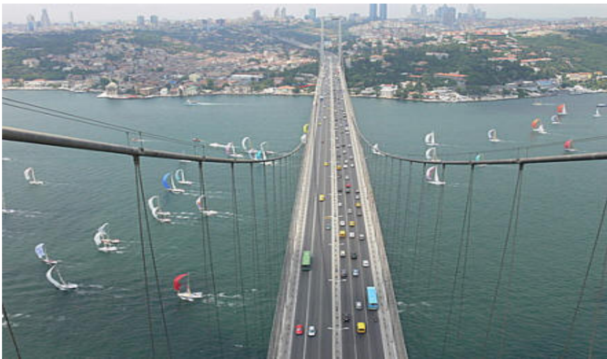
Bosphorus Bridge- Turkey
