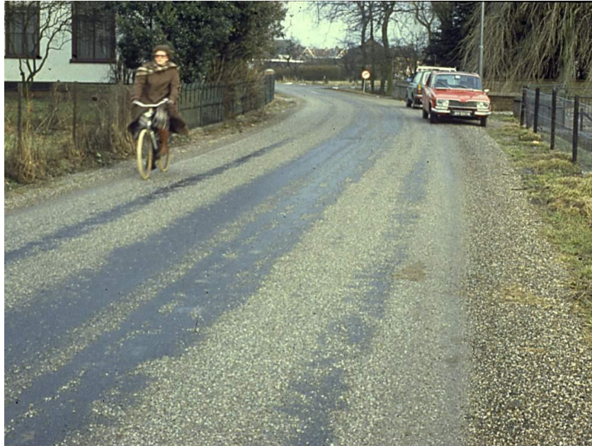
Figure 315: Raveling of a seal coat.
