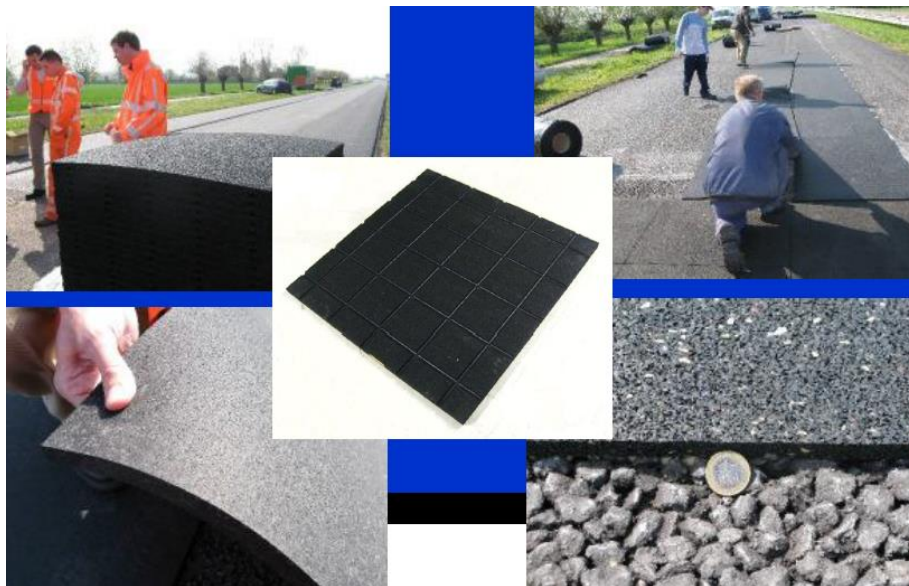
Figure 371: Construction of a PERS wearing course in the Netherlands.
