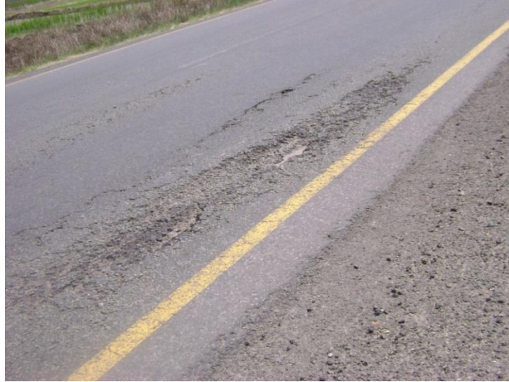
Figure 313: Raveling as observed on the TanZam highway.
