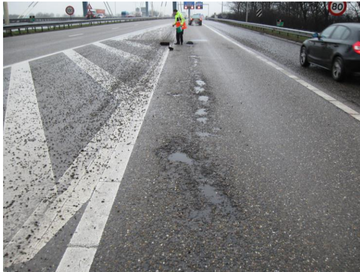
Figure 314: Raveling as observed on a porous asphalt concrete wearing course in the Netherlands.
