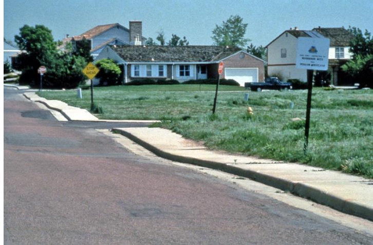
Figure 389: Unevenness due to an uneven swelling clay subgrade.
