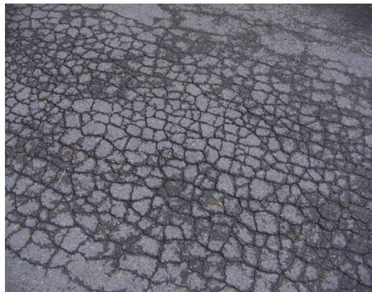
Figure 186: Example of cracking due to aging/hardening of the binder.
