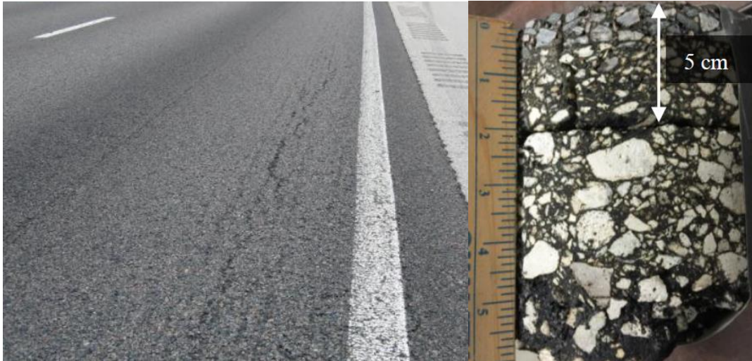
Figure 301: Cracking in wheel path limited to the wearing course probably due to loss of adhesion between wearing course and underlying structure.
