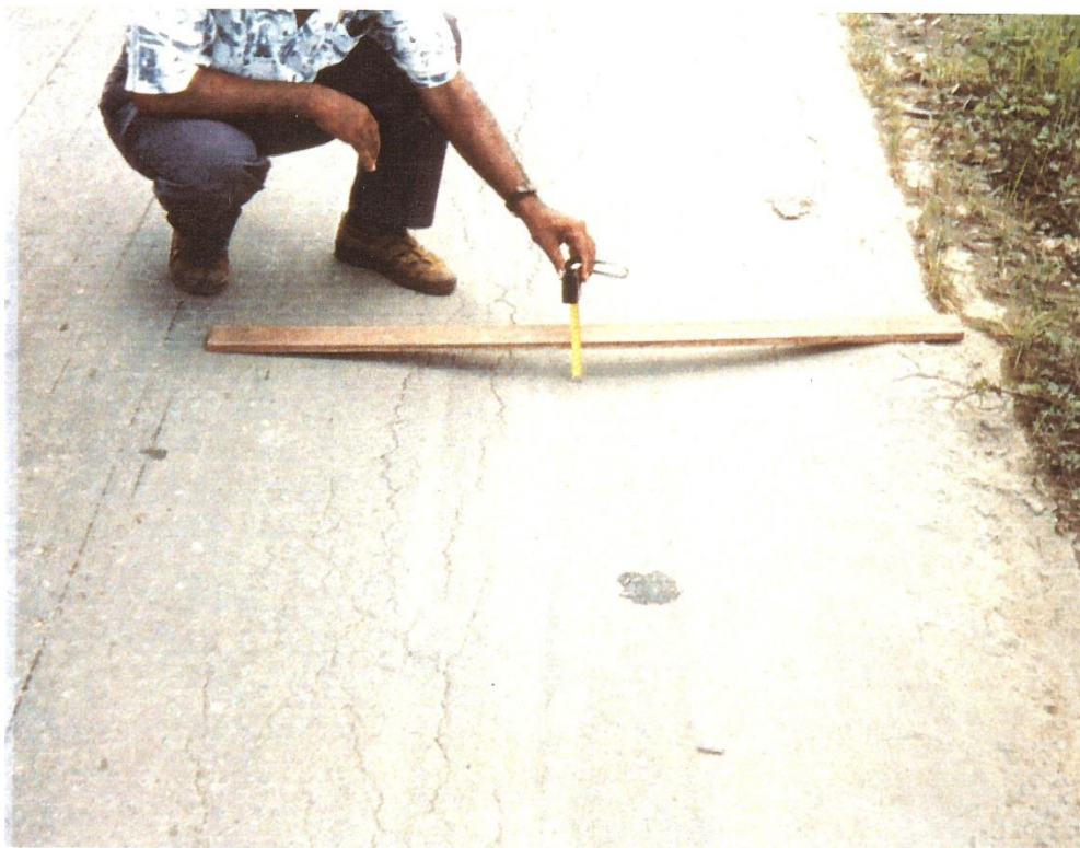
Figure 220: Excessive pavement deformation due to deformation of the unbound base and/or sub-base layer.
