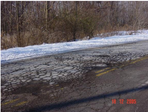
Figure 8: Roughness due to severe cracking.
