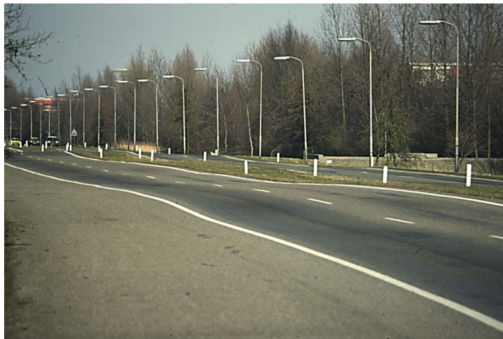
Figure 390: Unevenness due to uneven settlement of the weak subgrade.
