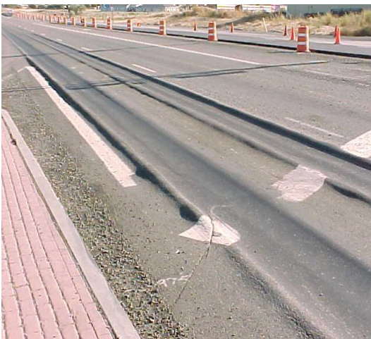
Figure 11: Rutting in an asphalt pavement.
