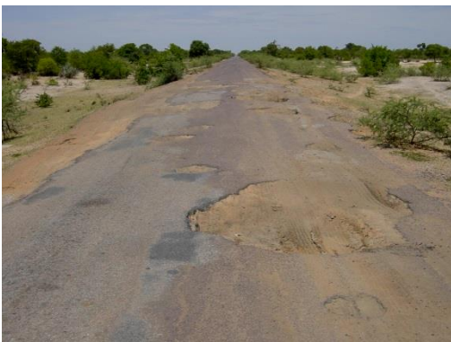
Figure 8: Roughness due to severe cracking.
