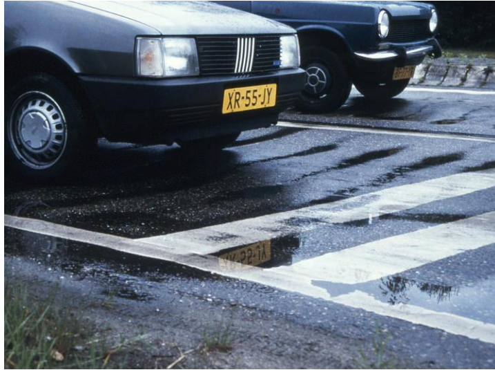
Figure 387: Corrugations, also called washboards, at a traffic light controlled junction.
