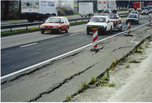
Figure 7: Severe longitudinal cracking due to shear failure in the existing embankment as a result of widening the road (extended embankment is on the right hand side).
