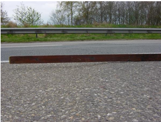
Figure 12: Unevenness due to “buckling” of the base made of blast furnace slag.
