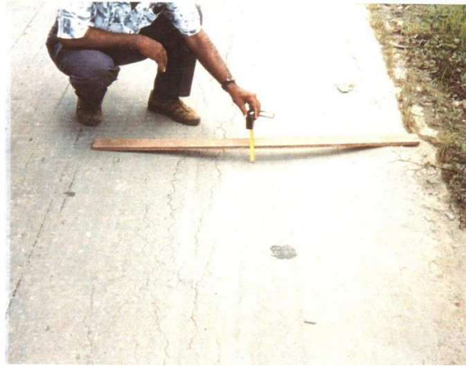
Figure 125: Permanent deformation caused by deformations in the layer(s) below the asphalt layer. Note the cracks!
