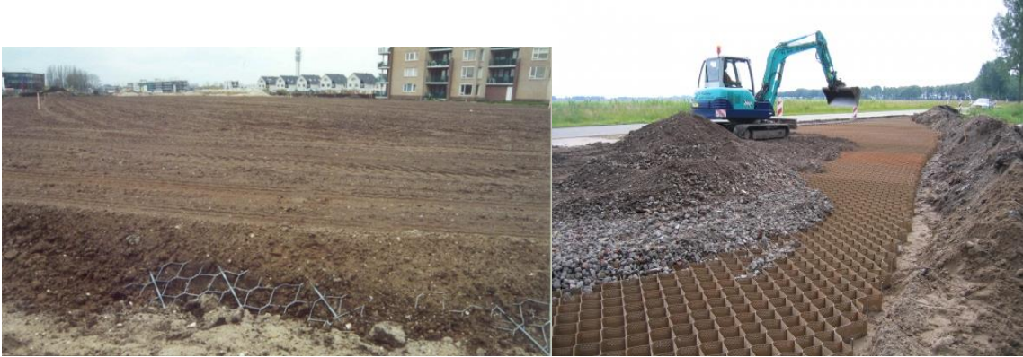
Figure 290: Use of reinforcement in unbound layers to provide confinement and reduce the amount of permanent deformation.
