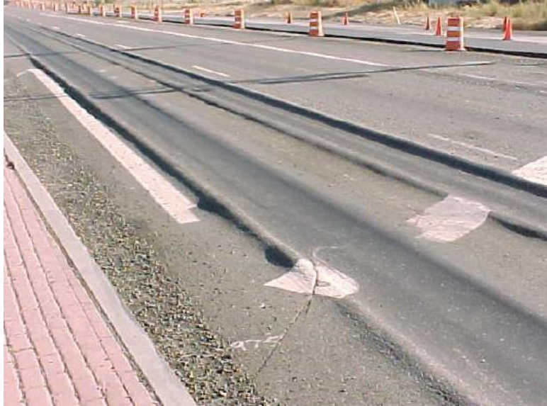
Figure 188: Permanent deformation in the asphalt layer.
