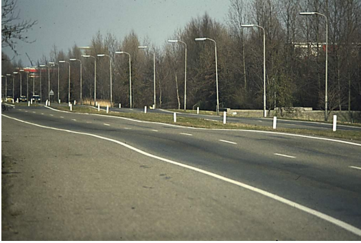
Figure 10: Longitudinal deformations due to settlements.
