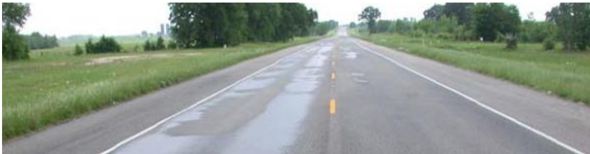
Figure 316: Bleeding observed on a road in the USA.
