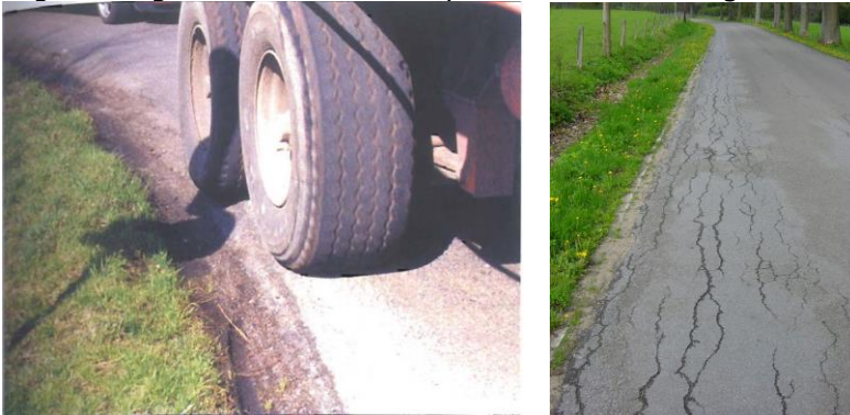
Figure 256: Edge loading and its consequences.
