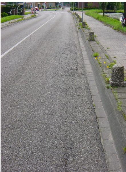
Figure 2: Longitudinal and alligator cracking in the wheel paths
