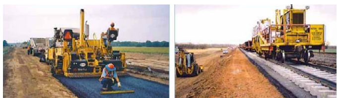
Figure 22. Placing asphalt sub-ballast (left) and the new track prior to adding the ballast and pulling the track up on the BNSF Railway 'transcon' capacity improvement project
