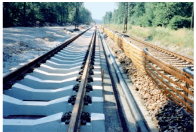
Figure 13. Two examples of SATO system: with Y-sleepers on asphalt (top) and concrete sleepers (bottom)
