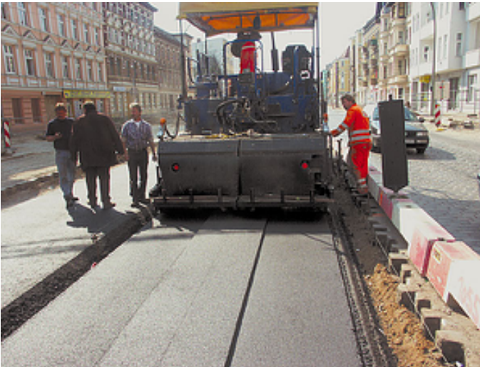
Figure 14. A paver with a special profile screed paving the top layer for the ATD-system to hold the sleepers in place later on [Source Voegele]
