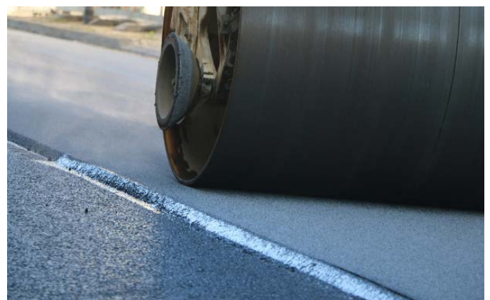
Figure 1. Compaction of asphalt layer
