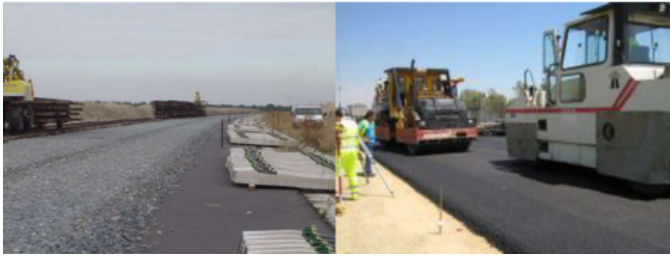
Figure 18. Bituminous sub-ballast sections built on the high-speed line Madrid-Valladolid, section between Segovia and Valdestillas (left) and on the high-speed line Barcelona-French Border, section Sils-Riudellots (right) [54]
