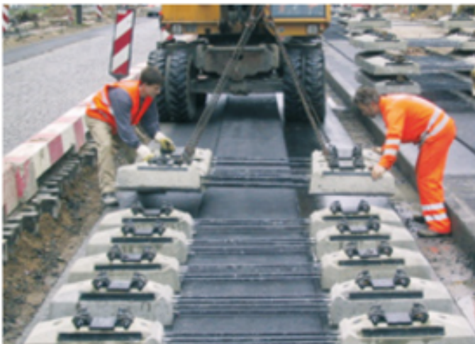
Figure 15. Placing the sleepers on the completed asphalt supporting layer [51]
