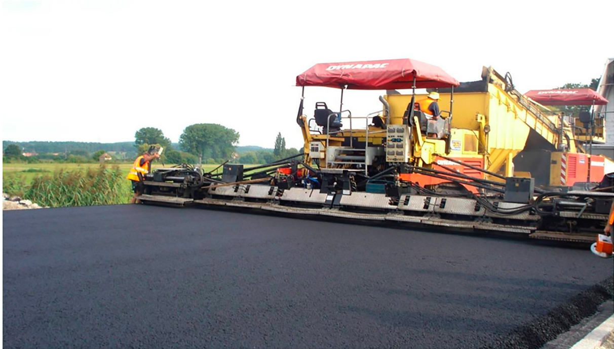
Figure 2, Laying of a SMA binder course
